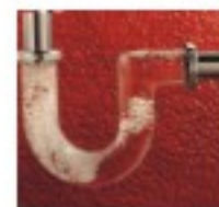
Organic waste collect on traps causing pipe blockage.
